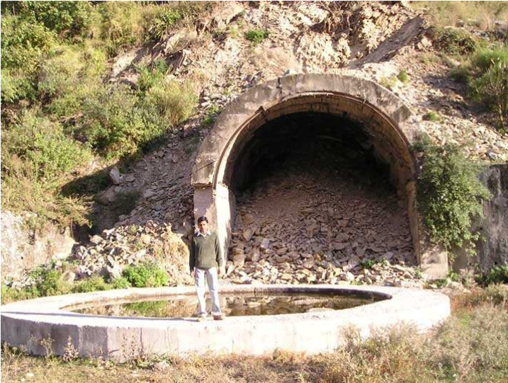
Photograph 4: abandoned tail-race tunnel near Nathpa.
